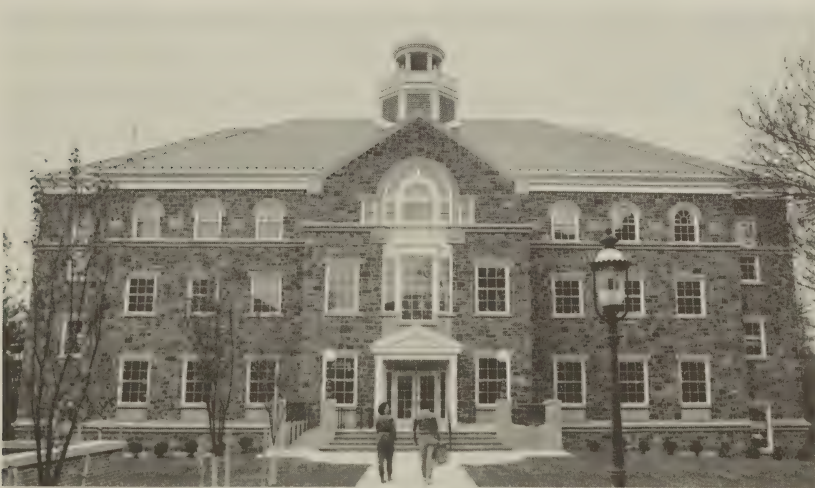
Templeton Hall – Completed 1989
